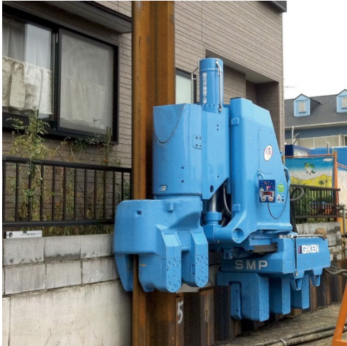
Zero Clearance Method
